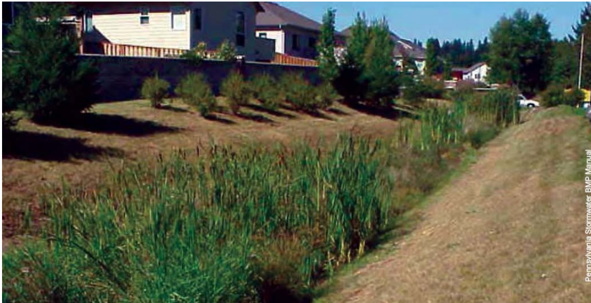
SWALE IN EASEMENT OF SUBDIVISION
